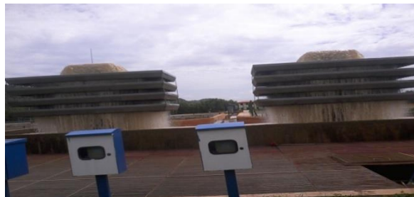
Figure 2.6: The cascade aerators
