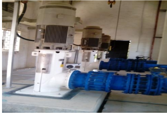
Figure 2.8: The Backwash Pump
