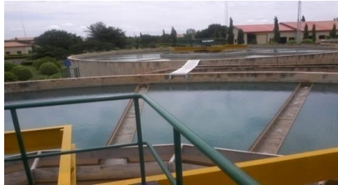
Fig.2.13: The Clariflocculator
