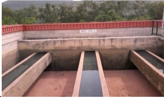
Figure 27: Gravity filter
